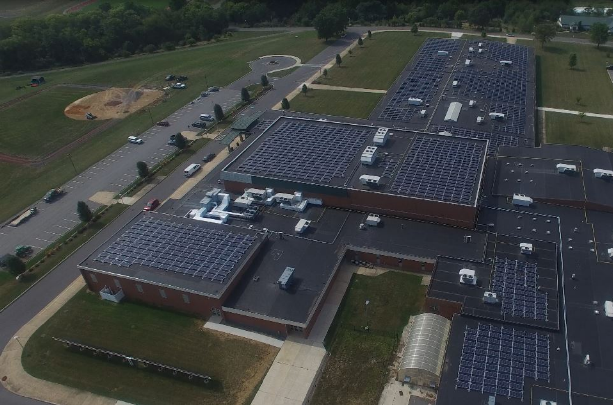
James Buchanan High School Rooftop Array
