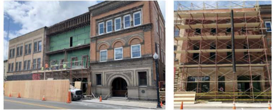
The existing building, pictured in the middle, had been vacant since 2015.
