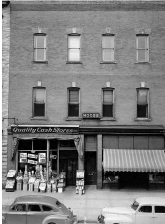
Historic photo of the existing building, circa 1930-1940.
